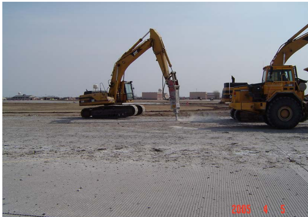
Figure 4.20. A ramhoe was used to further reduce the size of cracked PCC.
