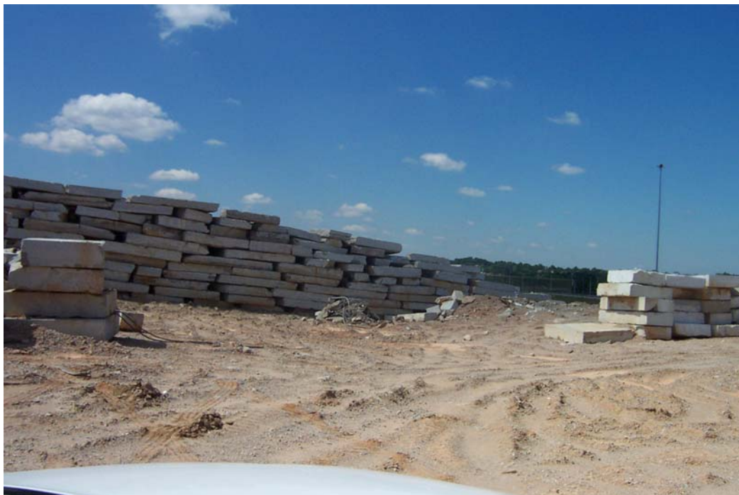
Figure 4.37. PCC slabs are stacked at ATL for future use as RCA.
