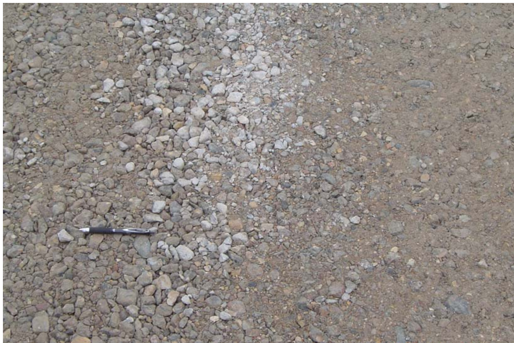
Figure 4.24. View of finished RCA base showing material segregation.
