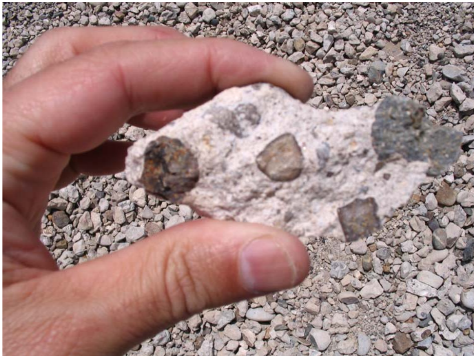
Figure 4.28. Condition of aggregate in parent PCC at Mountain Home AFB.
