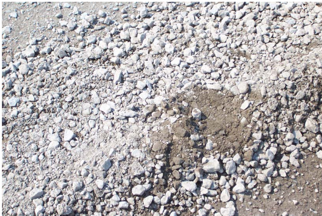
Figure 4.8. RCA material before compaction at North Auxiliary Field.
