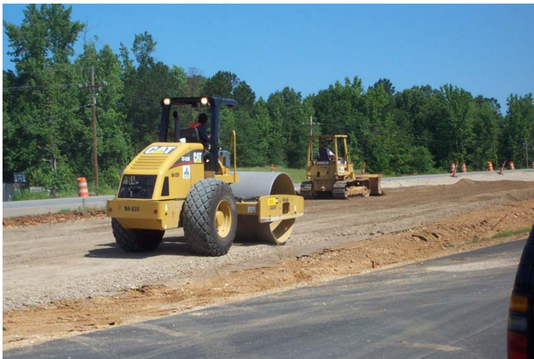
Figure 4.13. RCA being compacted using a vibratory roller at US 167.
