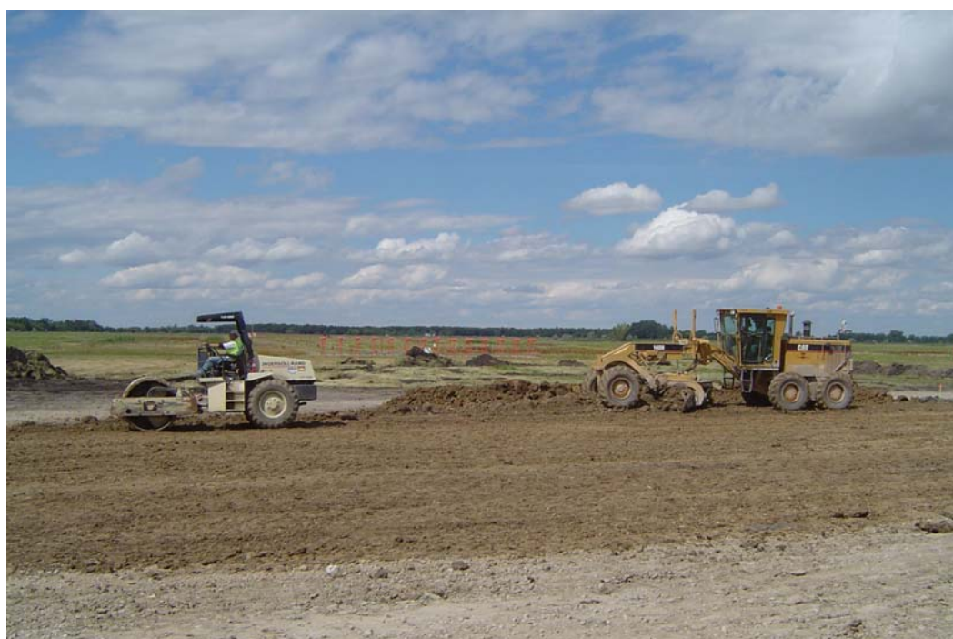
Figure 4.22. Subgrade preparation for Runway 17-35 at Grand Forks AFB.
