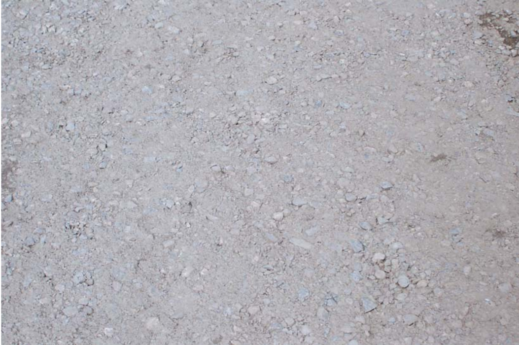
Figure 4.9. Finished RCA base surface at North Auxiliary Field Taxiway No. 2.
