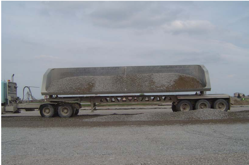
Figure 4.23. Plant mixed RCA base material was side dumped on finished subgrade.
