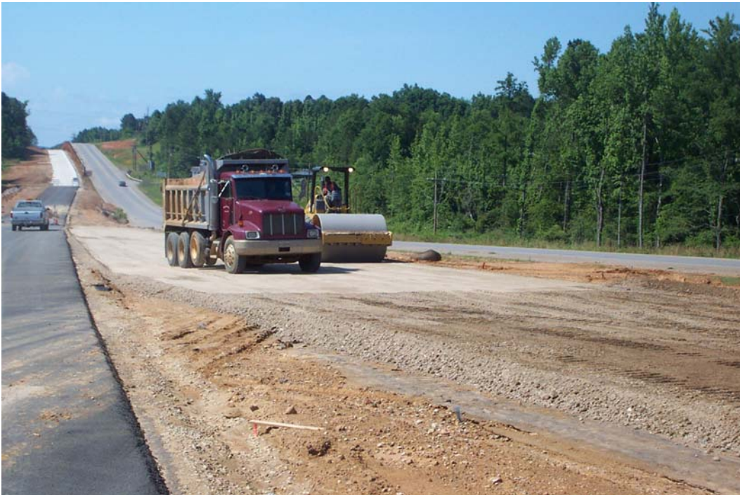
Figure 4.17. Construction traffic was allowed on compacted RCA base.
