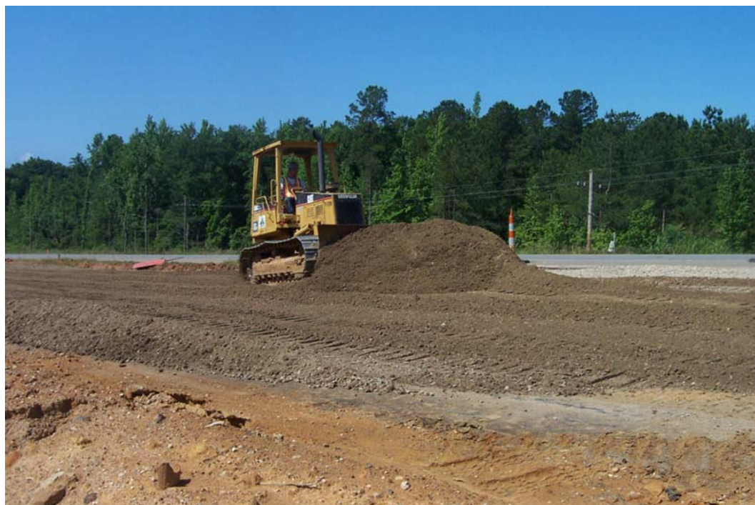
Figure 4.12. A bulldozer was used to spread RCA base material to grade.
