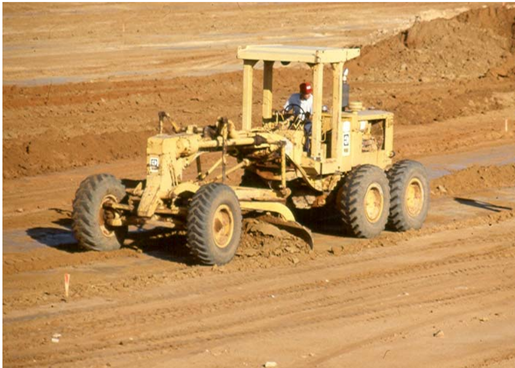
Figure 4.2. Typical subgrade preparation at Shaw AFB (Runway 4I-22R).
