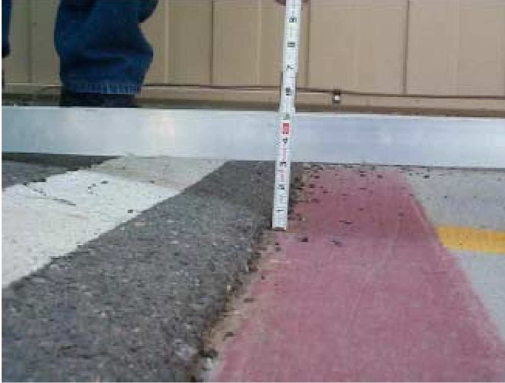
Figure A.29. Example of sulfate attack heaving on RCA base (Rollings et al., 2003).
