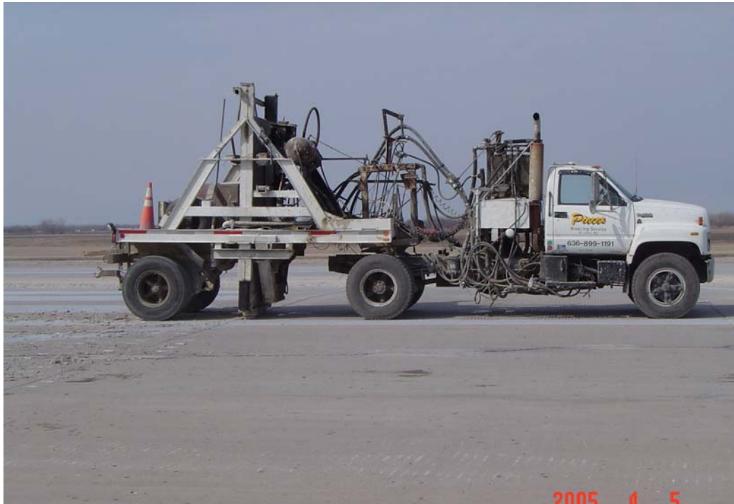
Figure 4.19. A guillotine was used to crack existing PCC at Runway 17-35.
