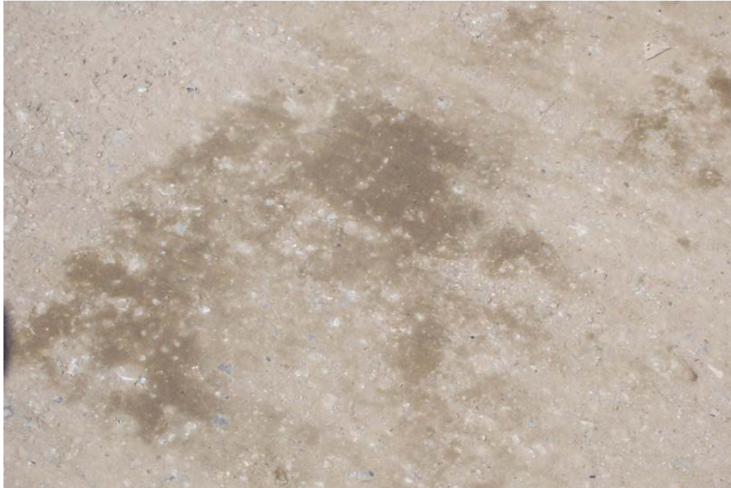
Figure 4.14. Typical RCA base surface after compacting at the proper moisture content.
