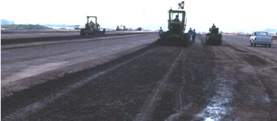
Figure 4.5. RCA base grading (motor grader) and compaction (rubber tire roller).
