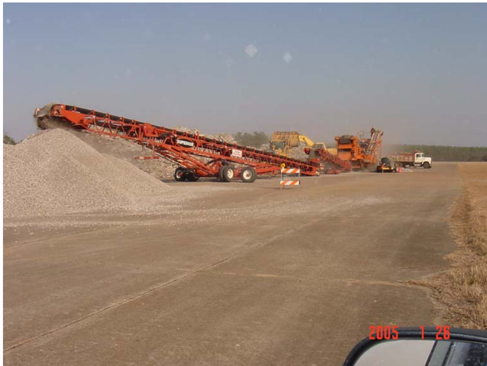
Figure 4.7. Crusher was set up on job site at North Auxiliary Field to produce RCA.
