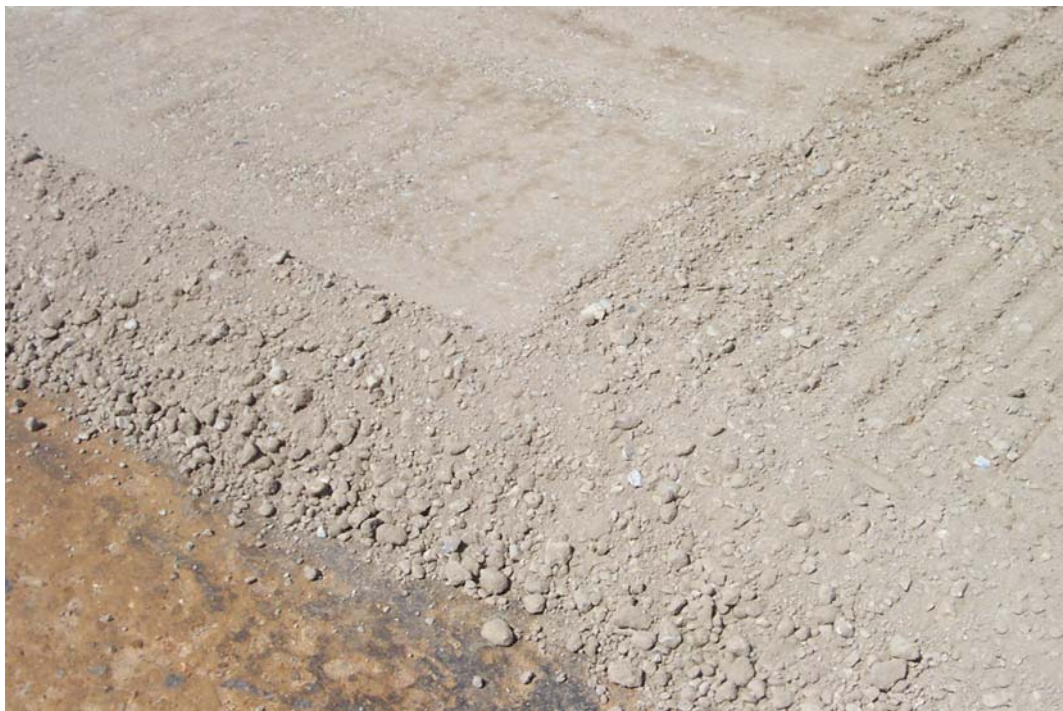
Figure 4.15. Typical RCA surface condition when further rolling should be avoided.
