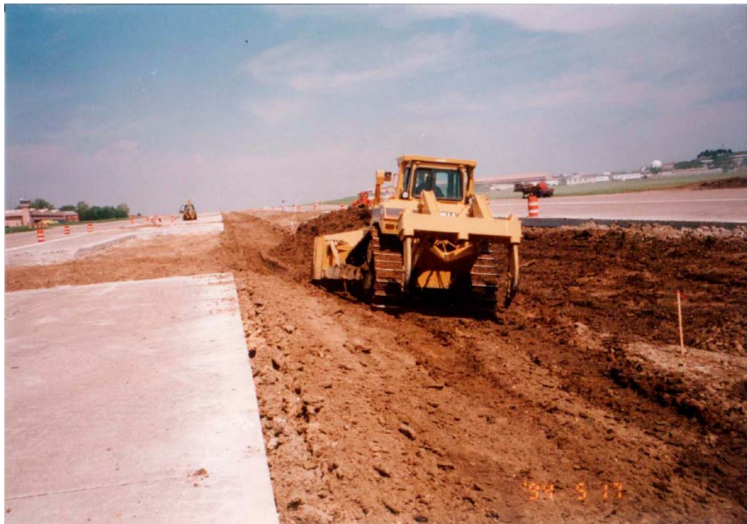
Figure 4.31. The keel section was excavated to a depth of 10 ft (10:1 side slopes).
