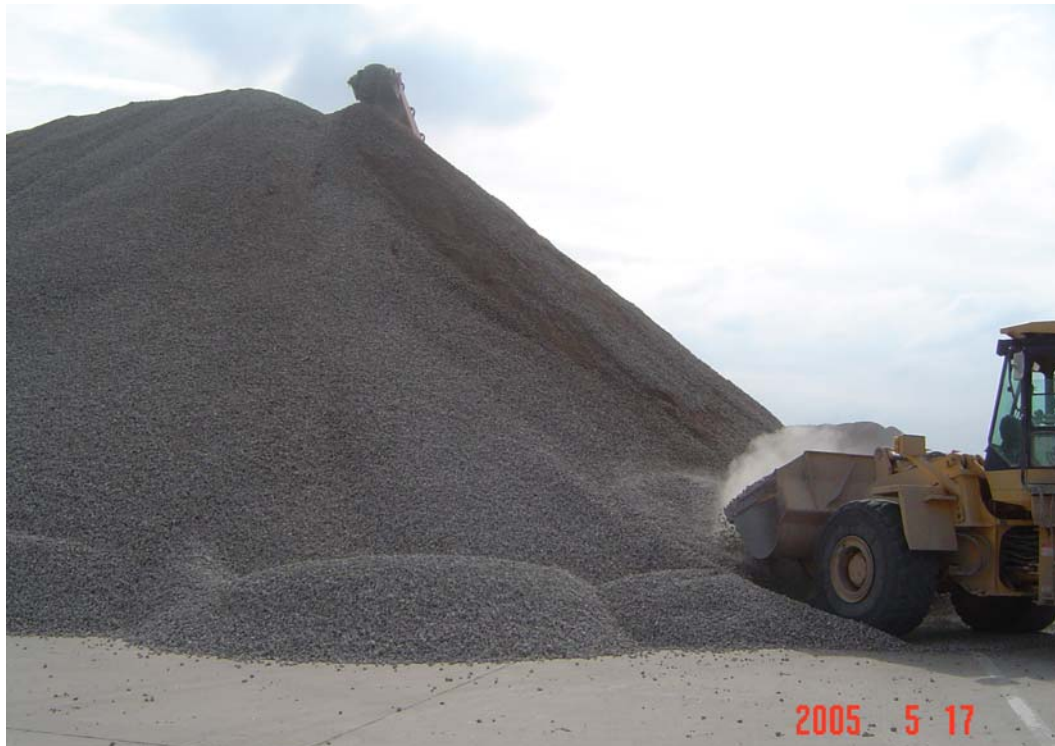
Figure 4.21. Crushed PCC material was stockpiled on site.
