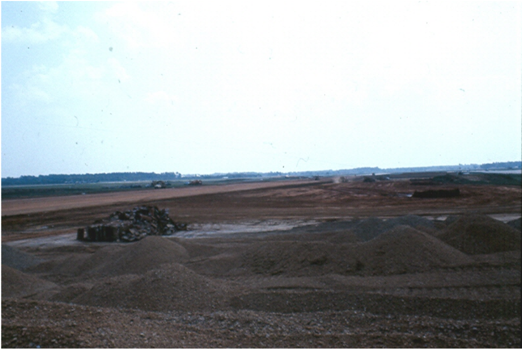
Figure 4.3. RCA was placed in windrows on prepared subgrade.
