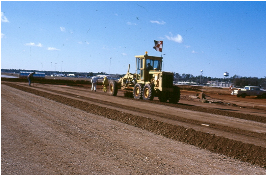
Figure 4.4. RCA was spread out to grade using a motor grader before compaction.
