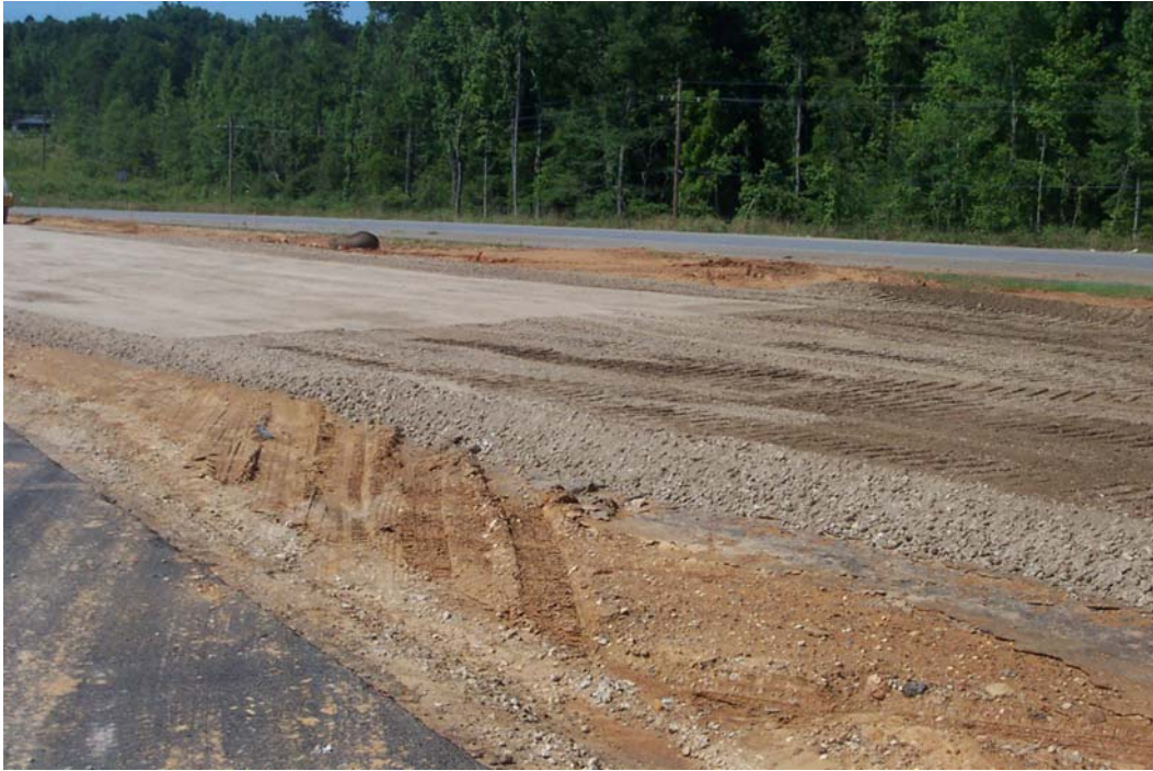
Figure 4.16. RCA base surface condition during proper spreading and compacting.
