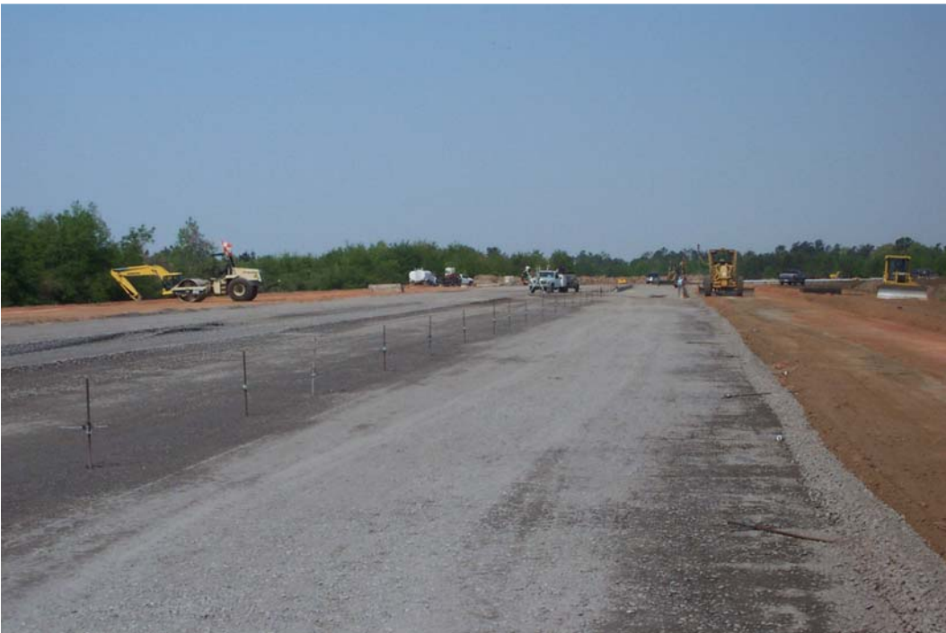
Figure 4.10. Construction of RCA base utilized standard construction equipment.
