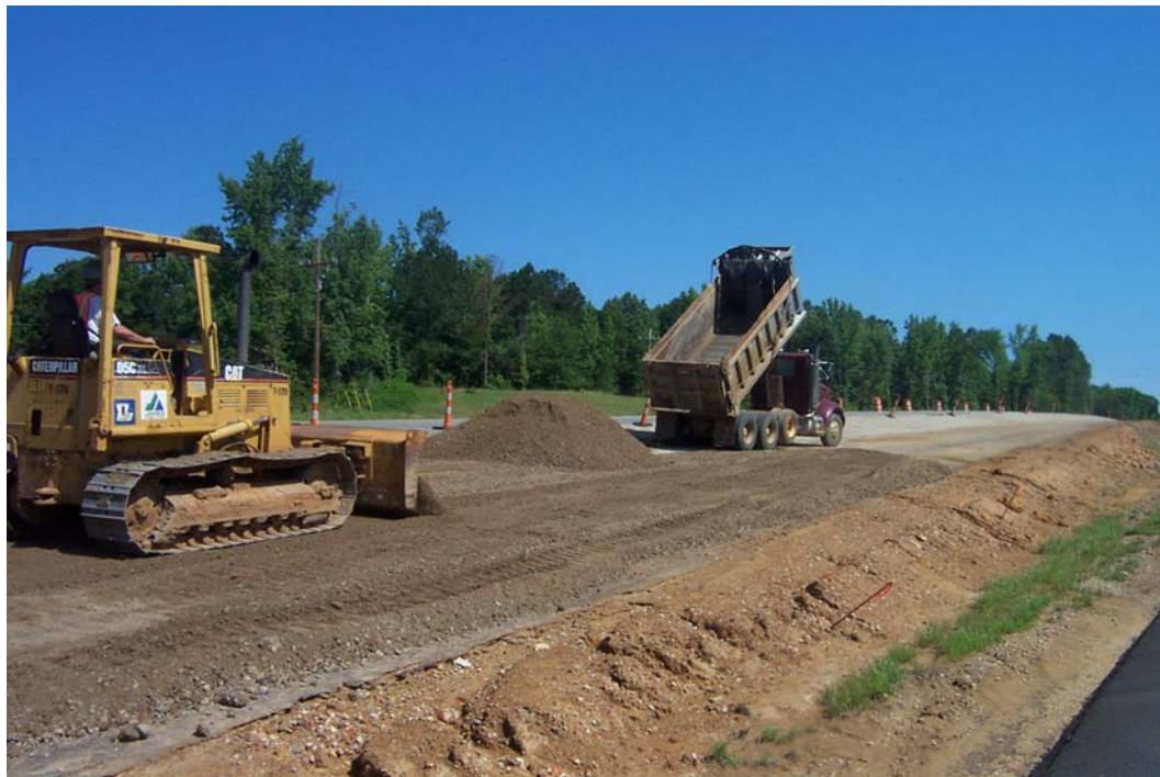
Figure 4.11. Construction equipment used for RCA base construction on US 167.
